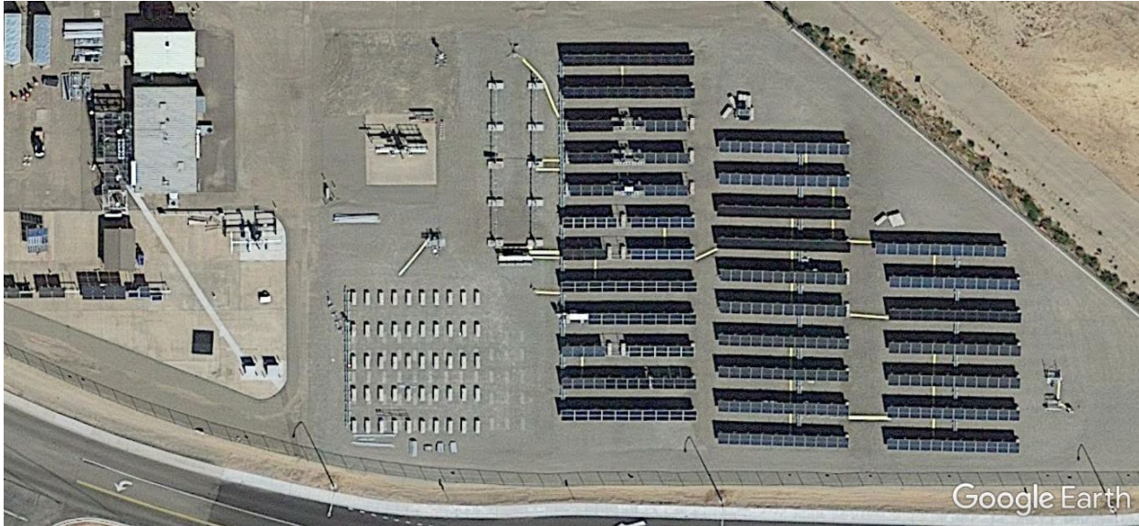
Figure 1 Site photo showing the location of PV the arrays. The dataset module temperatures are measured near the middle of the two middle rows in the middle section.
