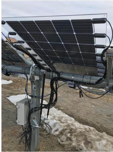
Figure 4 - Custom module with 12 individually addressable strings. Mounted in the middle of NREL's bifacial PV field.
